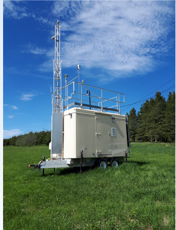
DELG's mobile air quality monitoring unit.
